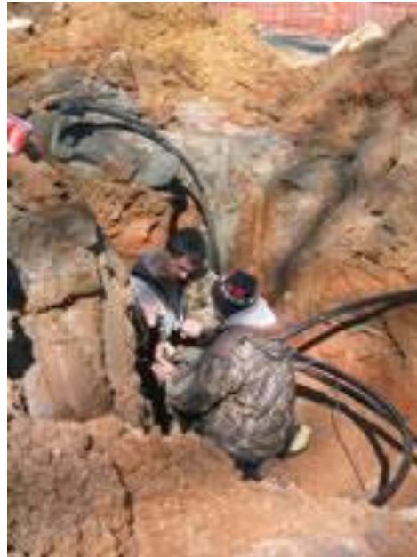
Ground Loop connecting well pipes and burying connections to house.
