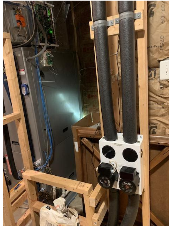
Well Pumps 1/6 hp
